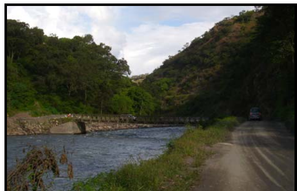
View of existing temporary Maranura bridge
