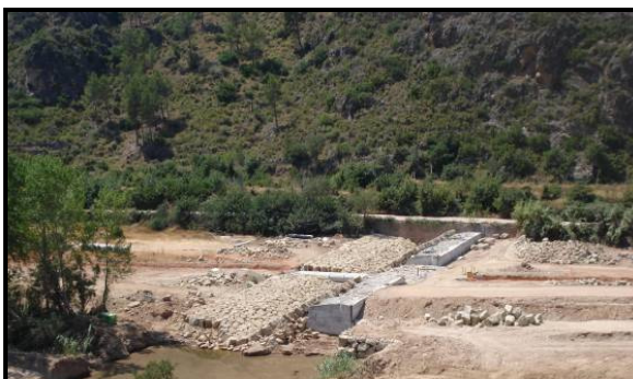
Dam 2 general view
