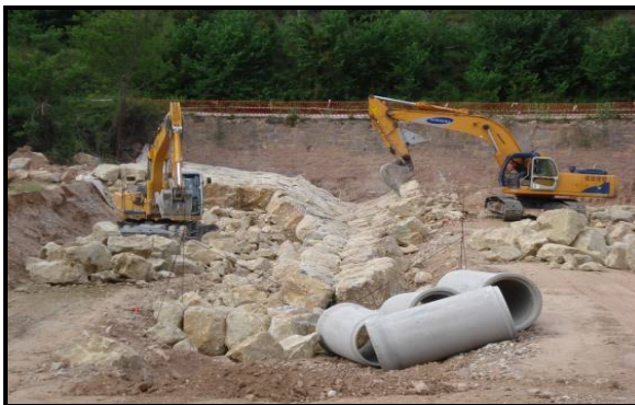
Breakwater basin Dam 2 buffering
