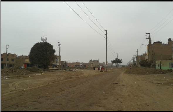
Current status of the road extension
